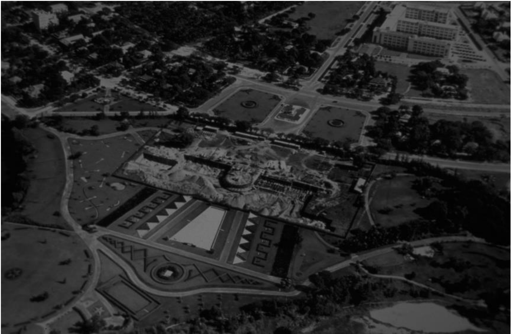
The building site of the new residence of the GG, ca. 1956
