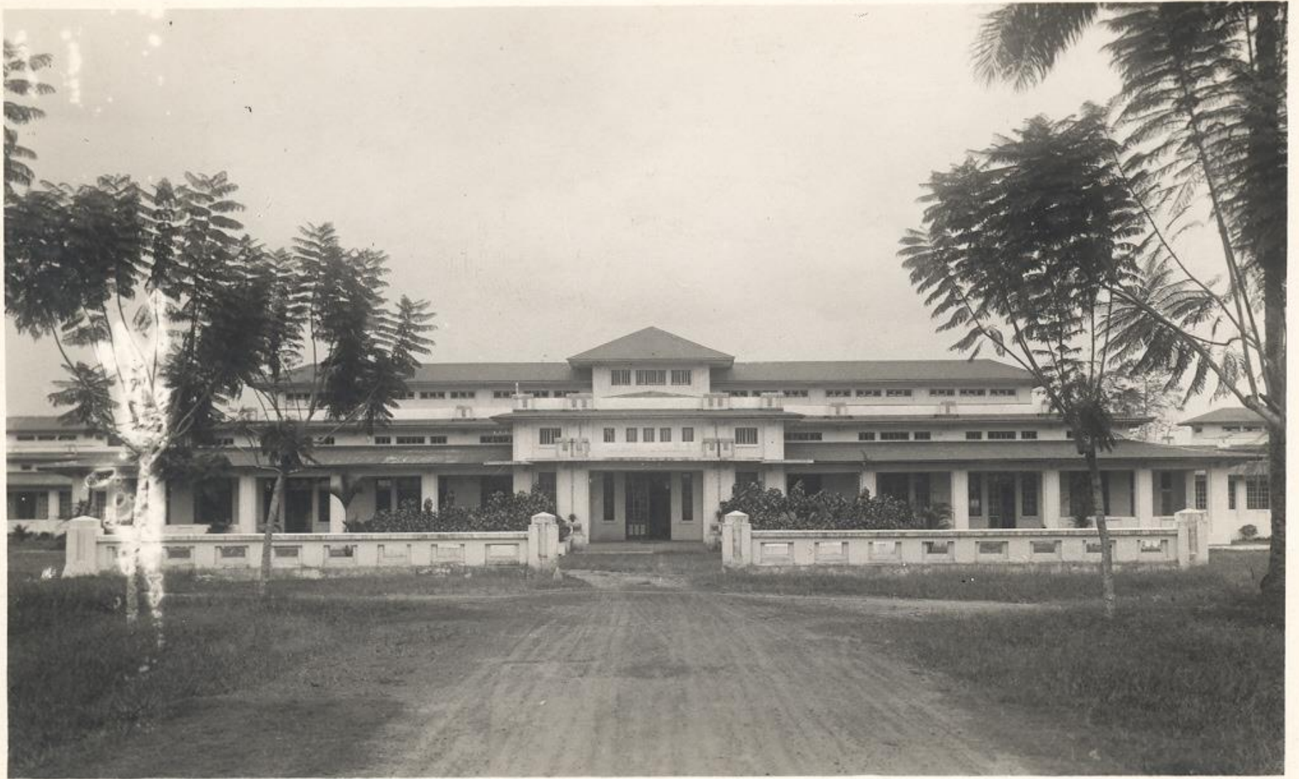
The colonial hospital for Europeans in Mbandaka, one of the “architectural jewels” of the city (provincial governor Duchesne)
